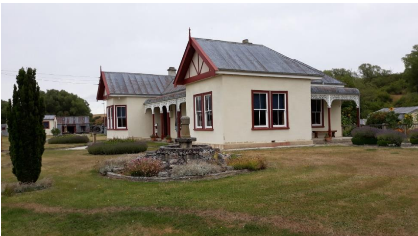
Historic Hayes Homestead at Otarehua
